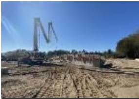
Port Stalashen Wastewater Treatment Plant
