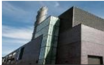
Markham District Energy
