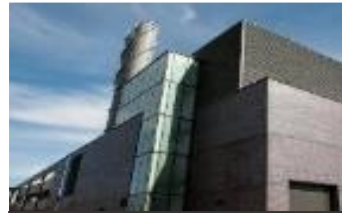
Markham District Energy
